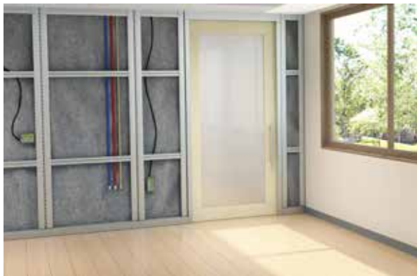
Water supply and now waste piping can be routed to the ceiling above.
